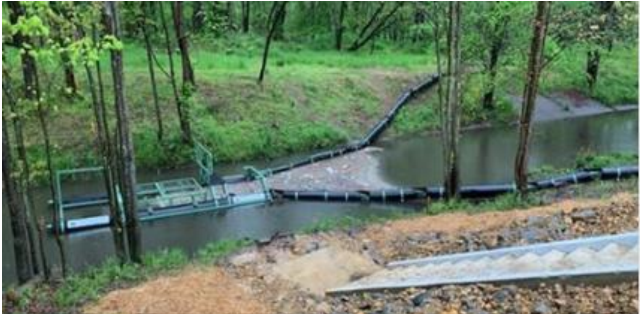
New trash trap in Little Hunting Creek
