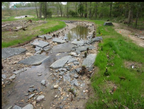
Examples of Natural Channel Design from the Wakefield Run Restoration
