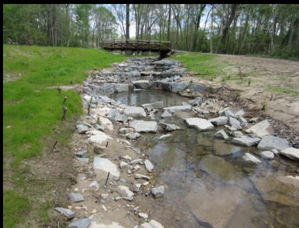
Examples of Natural Channel Design from the Wakefield Run Restoration
